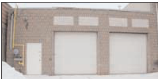
Rear Entrance/East Loading Doors
