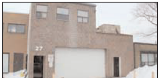
Main Entrance/ West Loading Door
